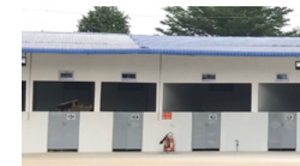
▲ Vietnam Plant 3 (Tan Phu) Waste Separation Storage
