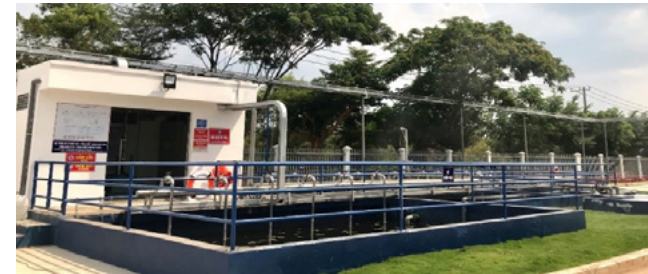
▲ Vietnam Plant 3 (Tan Phu) wastewater treatment plant
